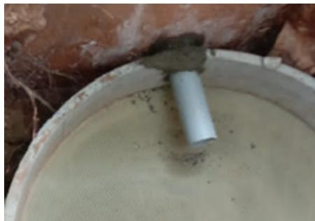
Soak tank with filter membrane
